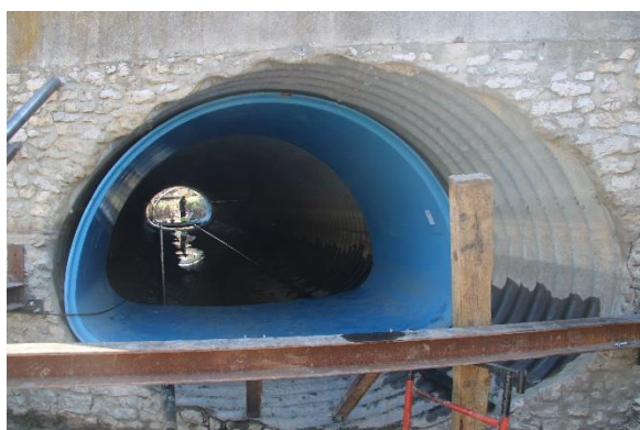
Figure 16b – Installation of the GFRP pipes.
