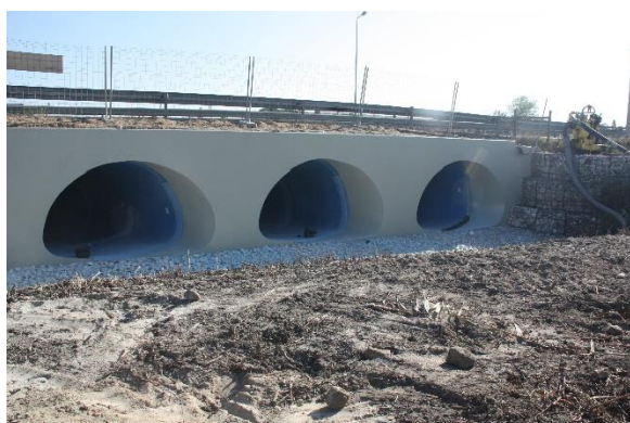
Figure 16d – PH after rehabilitation.
